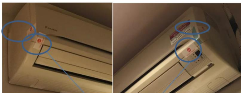
Warning labels at the air conditioner 冷氣機警告貼紙
